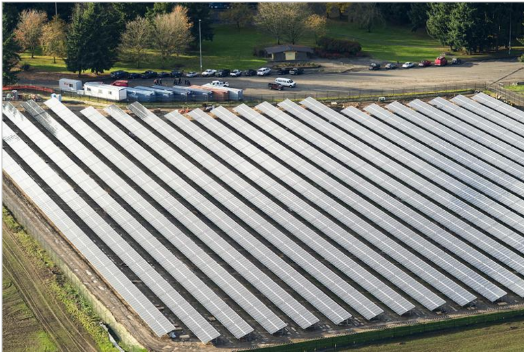
Figure 5: Aerial view of Oregon DOT's Baldock Safety Rest Area Solar Highway Project Photo credit: Gary Weber, Oregon DOT
