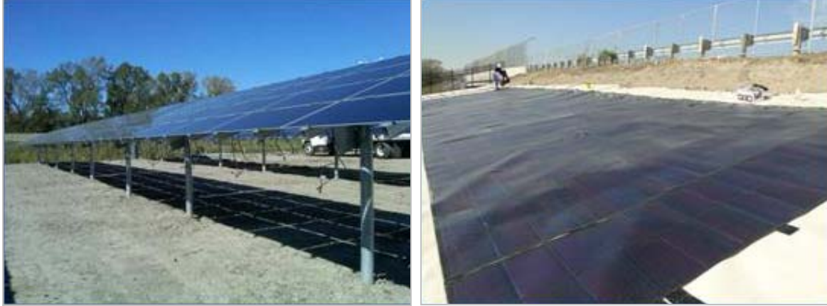
Figure 7: Rigid First Solar panels (left) and flexible Xunlight Corporation solar panels (right) installed along I-280 in Toledo, OH
